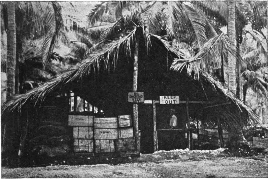
Figure 149. Covered storage constructed of local material.
